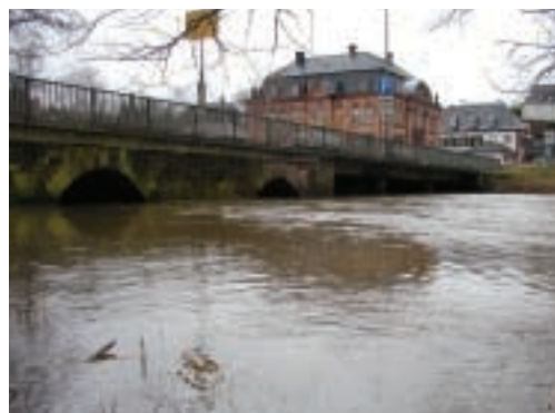
Source: Fotoshop Schmidt, Blieskastel
